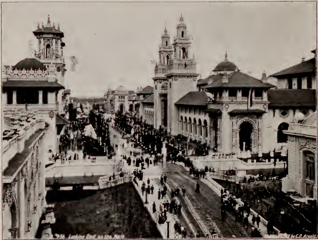
LOOKING EAST ON THE MALL.—The view gives a good idea of the Sunken Garden between the Machinery and Electricity buildings, and of the towers of Machinery, to the right, and Electricity, to the left, which, in their different ways, are notable examples of the Spanish Renaissance style.
